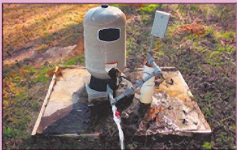
Domestic well, Early County, Georgia
