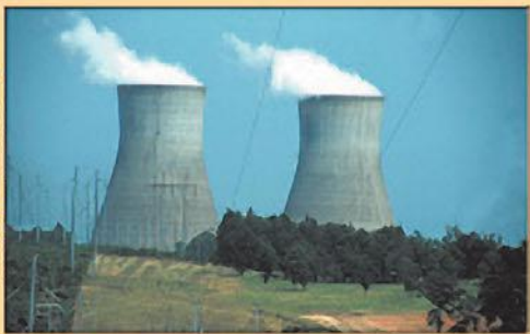
Cooling towers, Burke County, Georgia
