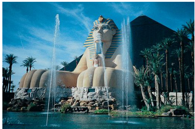
FIGURE 19.20 Water reuse at a Las Vegas, Nevada, resort hotel.
