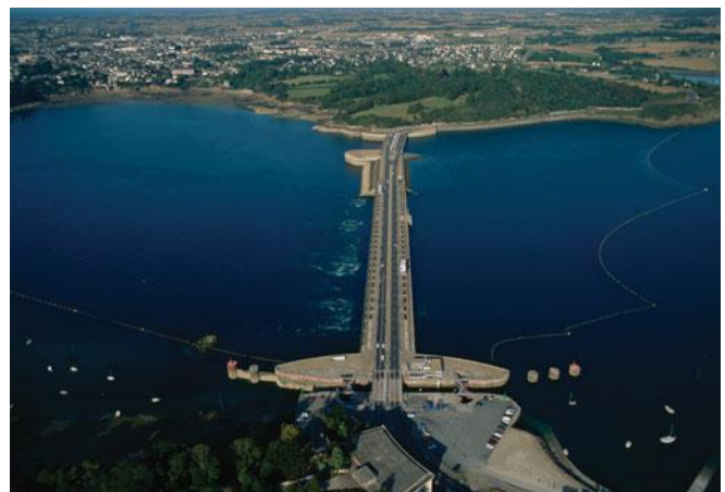
FIGURE 16.12 Tidal power station on the river Rance near Saint-Malo, France.
