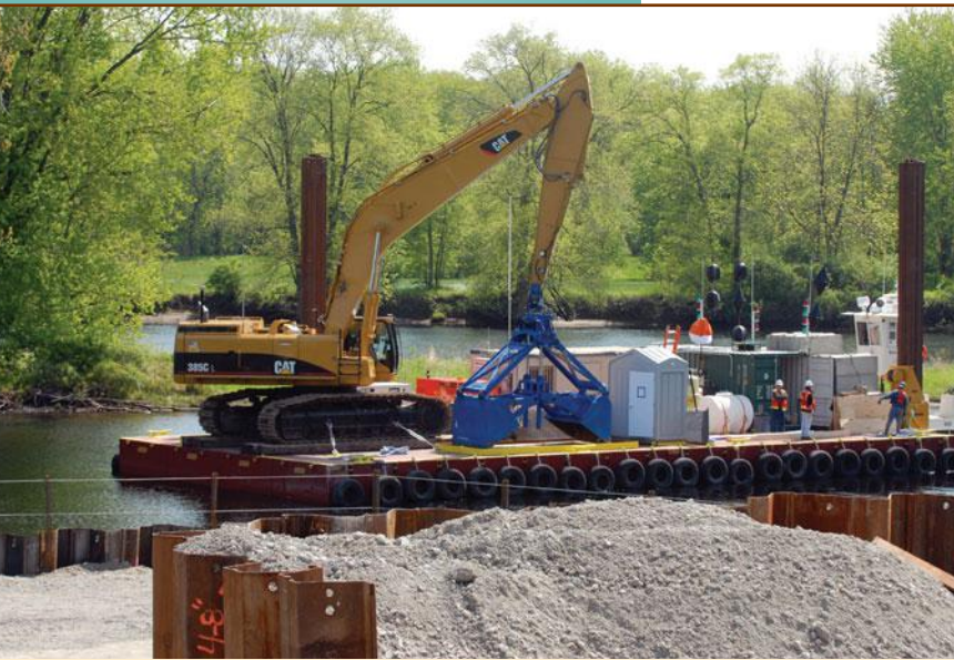
Dredging began in 2009 to remove contaminant sediment from the Hudson River in New York.
